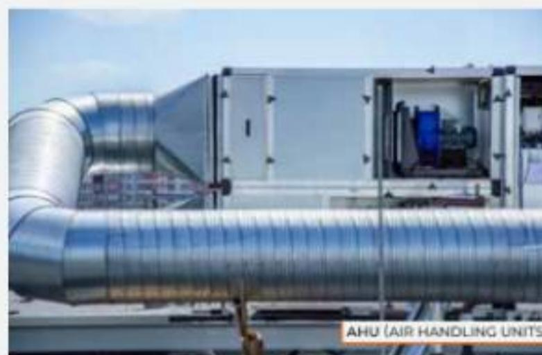
AHU (AIR HANDLING UNITS)
